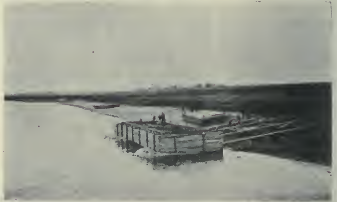
Fig. 4.—Launching caisson for pier No. 3.
